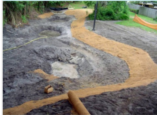
Figure 5. Stabilize the banks each day following excavation of a stormwater wetland.
