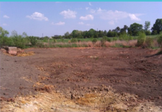
Figure 6. The soils for this stormwater wetland are properly prepared for water and wetland plants.
